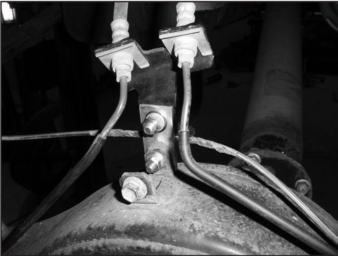
FIGURE 65A - LOOKING FROM BACK
